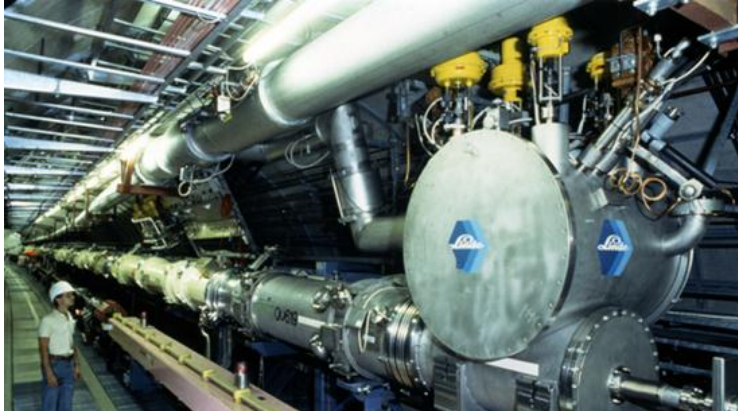
HERA feed box for cryogenics and magnet current
