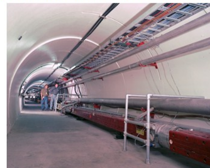
700 More Spare Tevatron Dipoles in the New Underground Magnet Storage Facility
