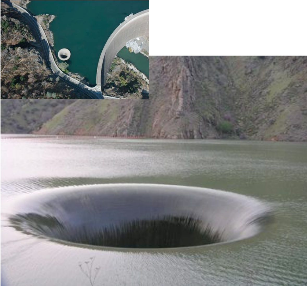
Bell-mouth spillway of Monticello dam, lake Berryessa, CA
