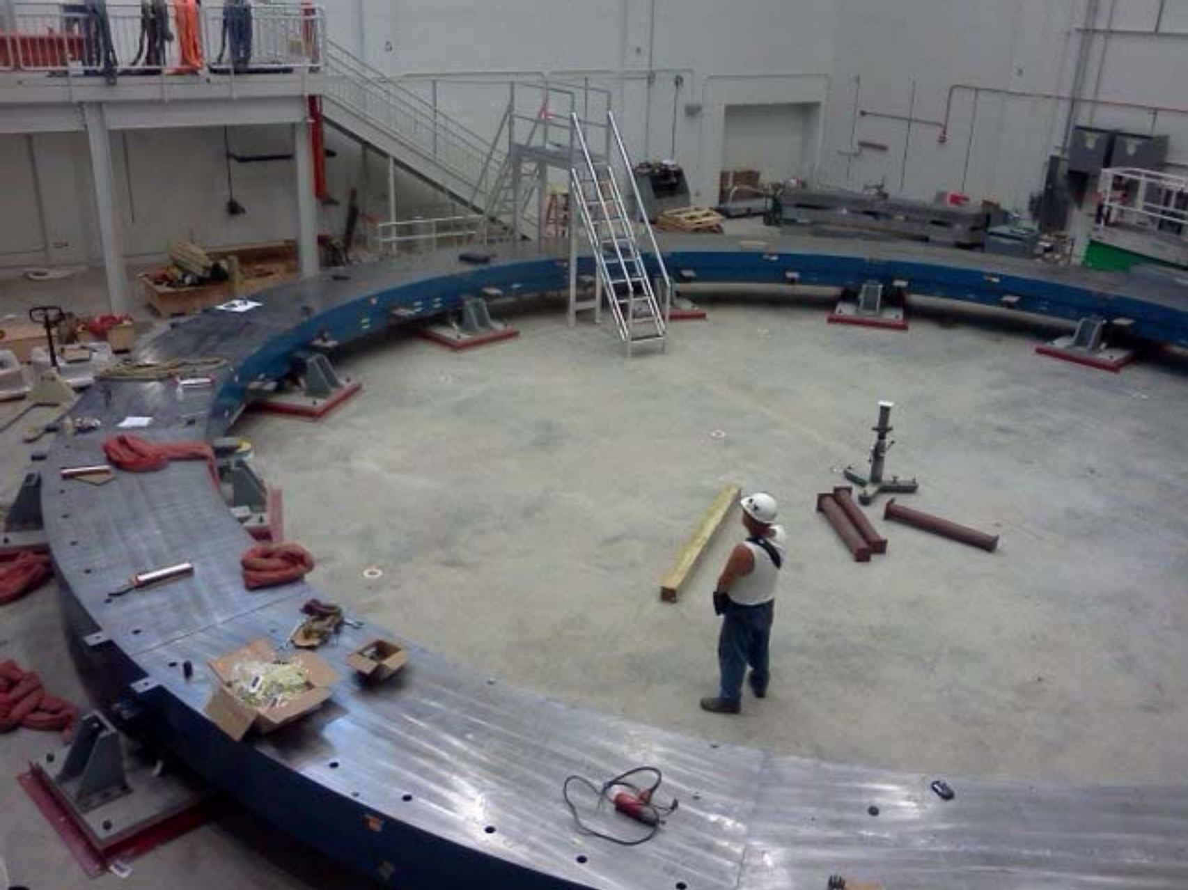
Bottom of magnet yoke being assembled at FNAL, June 26 2014
