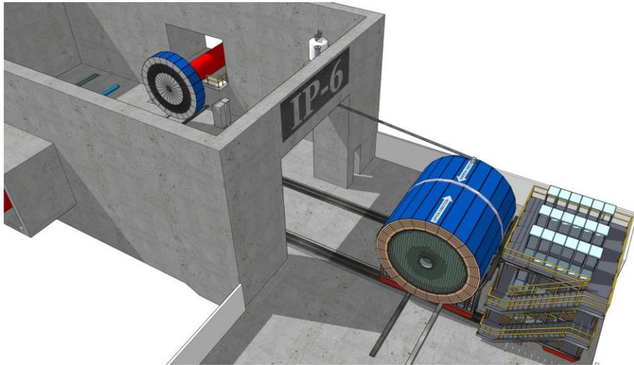
Image show how such a detector could be moved out of IP-6 at the EIC.
